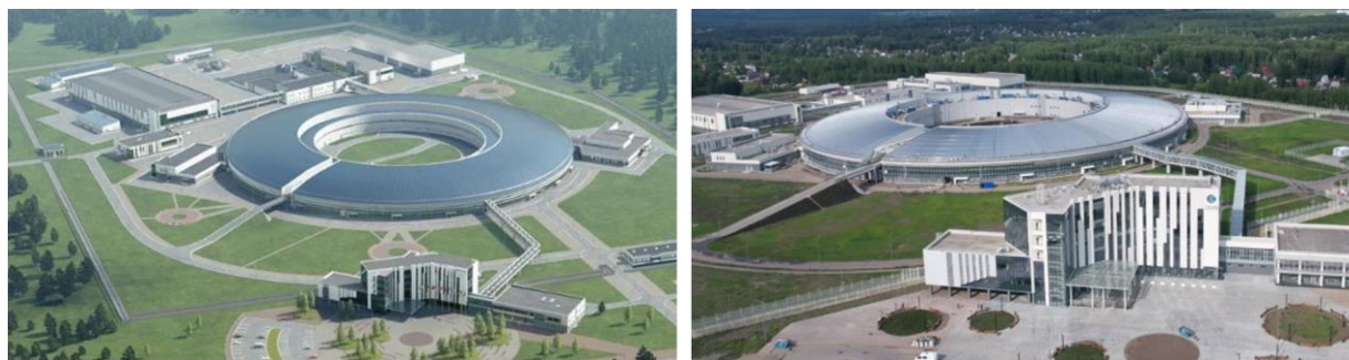
Fig. 1 Digital model of SKIF (left) and real aerial photo of the construction site as of mid of July, 2026
